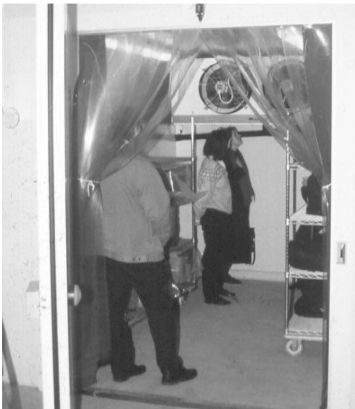
Figure 1. Purpose-built walk-in -30^{\circ}\text{C} freezer at the British Museum store.
