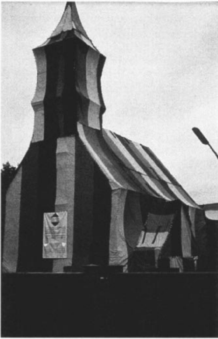
Figure 8.6 Church tented for carbon dioxide fumigation. (Photo courtesy of Gerhard Binker.)
