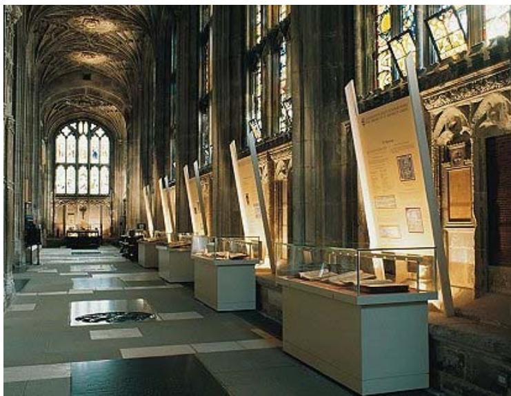
Fibre Optic Lighting: Gantry fitting giving an even spread of illumination - St George's Chapel Windsor Castle, Archive display
