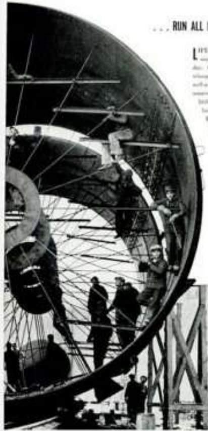
ALL RUN THROUGH THIS STEEL "LINER"
