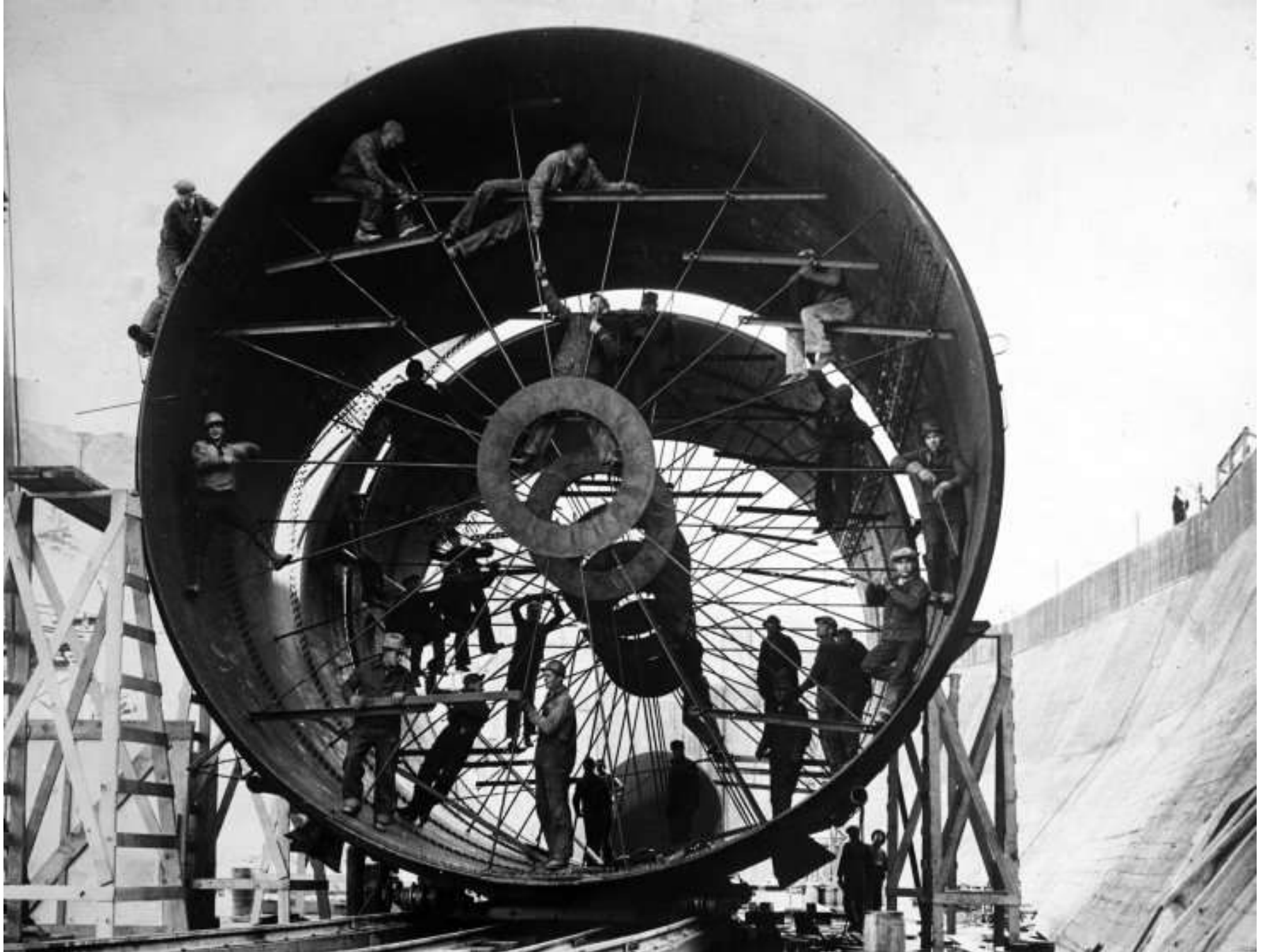
1/4 of Missouri River will run through this liner
