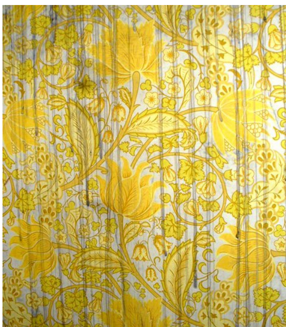
Figure 3 (above). Paper in the 3 rd floor corridor, exposed by removal of ducting, is very poorly attached to the wall. Figure 4 (left). Wallpaper from room 2.023 showing vertical staining pattern.
