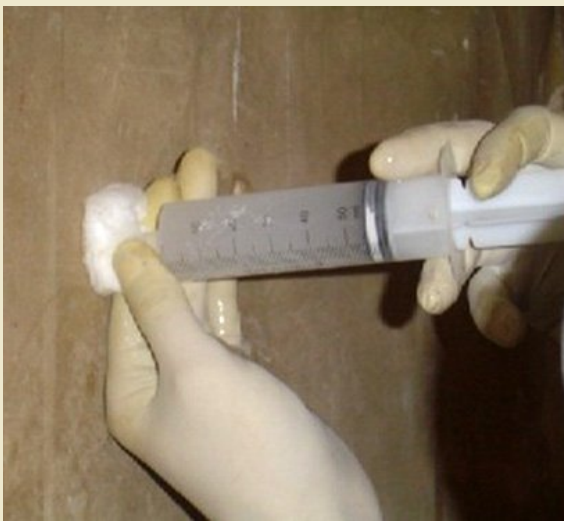
Figure 13. The grouting process started by making very small holes.
