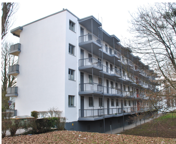
Walter Gropius building in Dammerstock, 2013.
