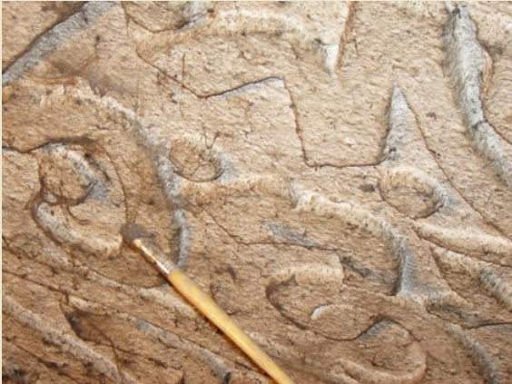
Figure 10 (top left). Cleaning new plaster and removing friable dirt's by using different sizes of soft brushes.
