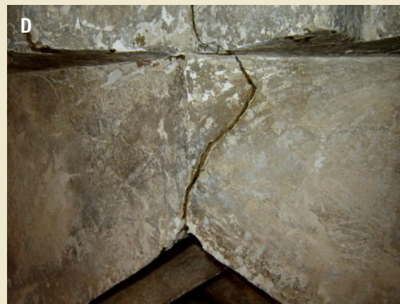
Figure 15. Restoration of the stalactite cracks: a) linen impregnated in primal AC33; b) compressed the linen rods inside the crack by spatula; c) linen inside the crack; and d) the surface covered by mortar layer.
