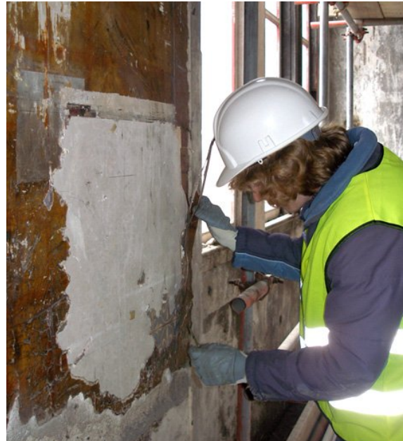
Figure 2. The author retrieving a fleur-de-lis style wallpaper from the 2 nd floor of the building.
