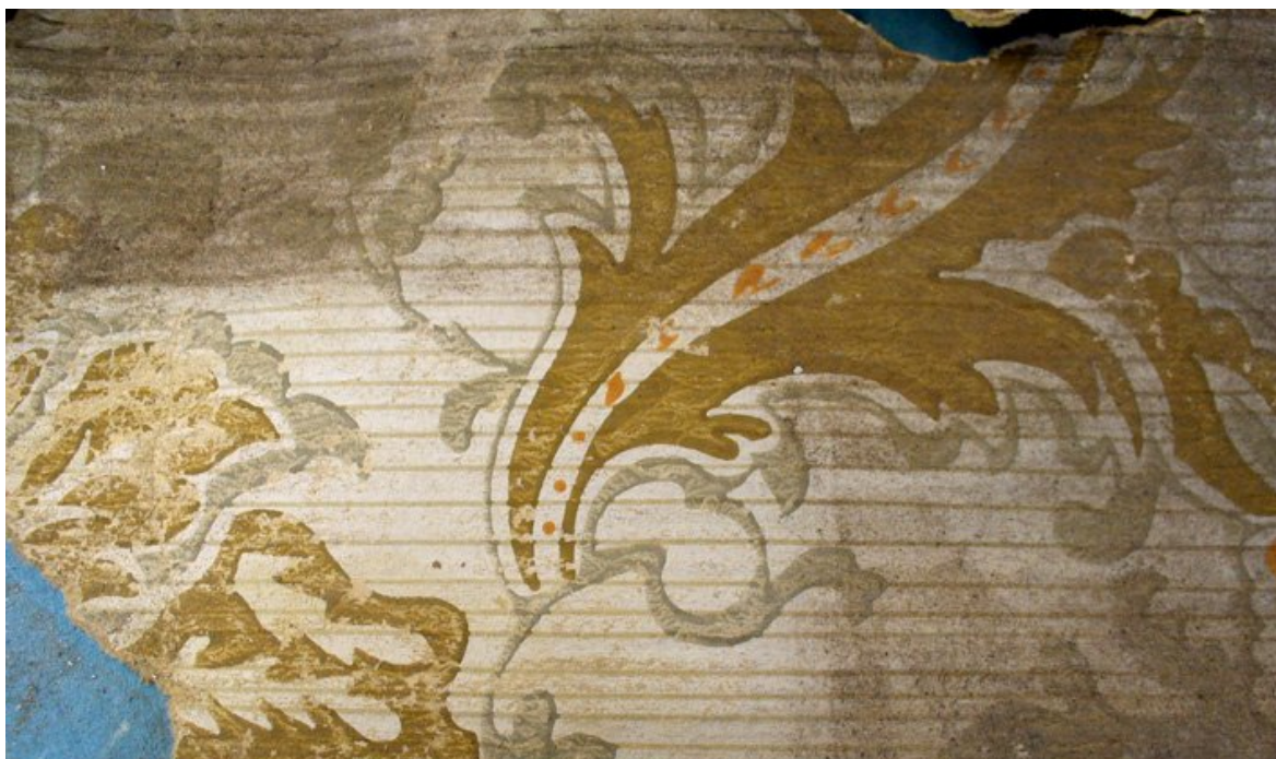
Figure 6. Using a smoke sponge for dry cleaning of wallpaper. The area bottom left of the photograph has been cleaned with a smoke sponge. The remaining areas are uncleaned.
