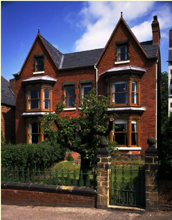
Figure 1. View of Mr Straws House. Mr Straws House is the righthand half of the semi-detached property, the property on the left is a visitor centre and exhibition space. ©National Trust Images/Rupert Truman
