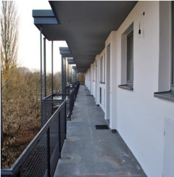
Walter Gropius building in Dammerstock, 2013.
